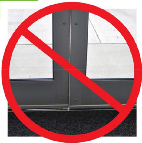
Standard aluminum pairs of doors leak air and water.
